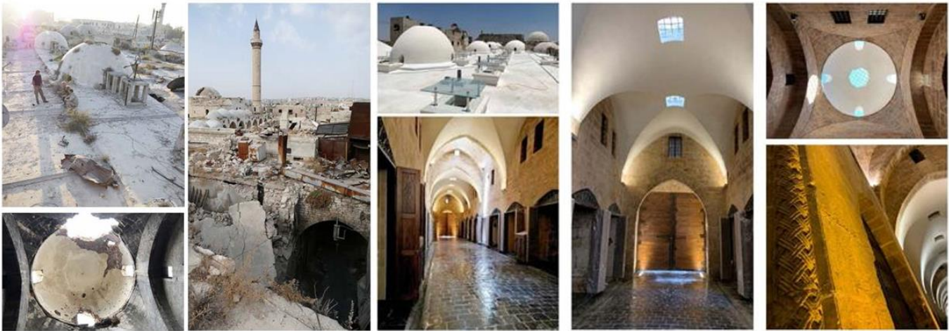
Figure 10: Souk al-Saqatiyya rehabilitation [60].
