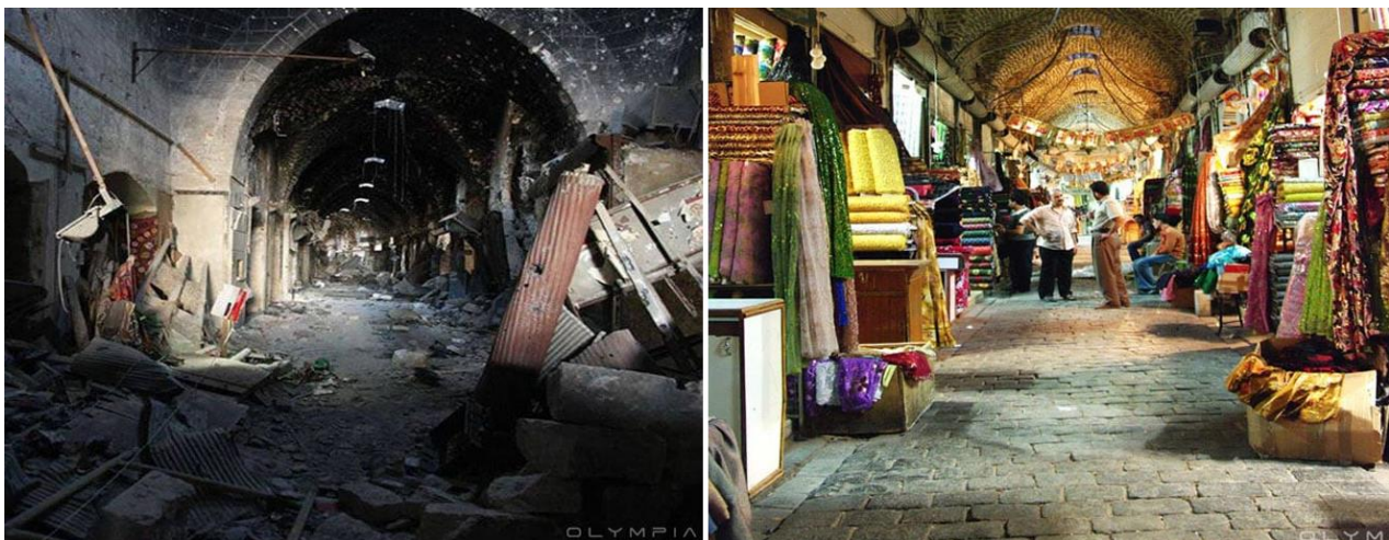
Figure 8: The damage in Aleppo's Old Souks before and after the war [58].
